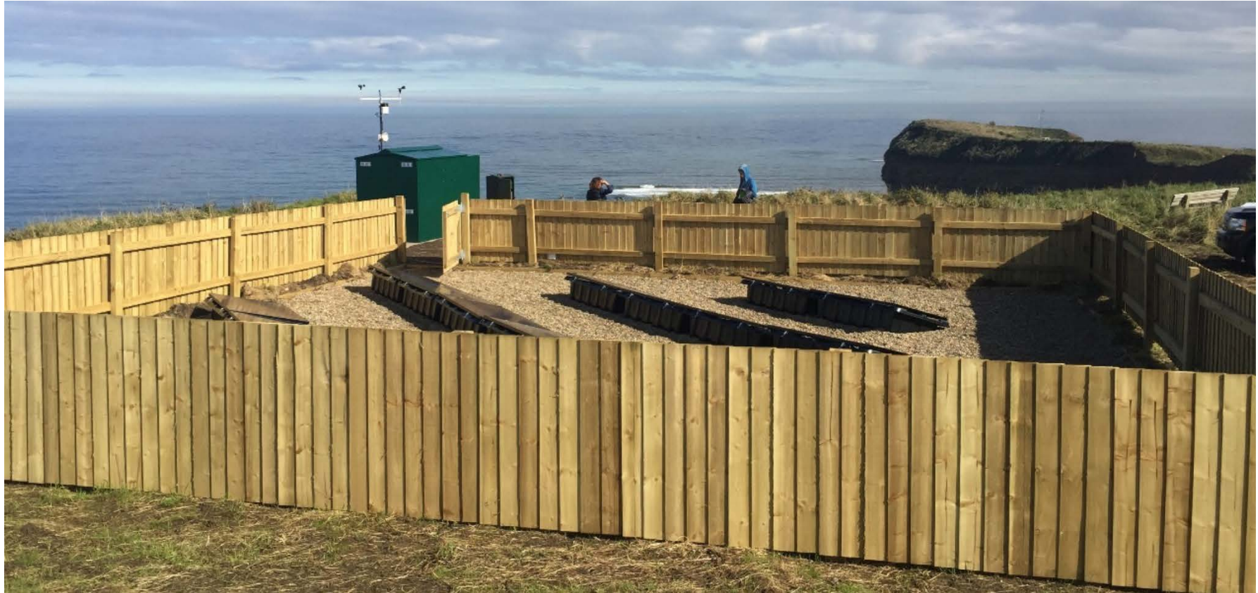
Figure 1. Completed installation of the fixed monitoring system at Cowbar Nab. In the foreshore is the solar power enclosure, providing off-grid power to the monitoring system. The larger green shelter houses the power control system, and the small green enclosure the monitoring instrument.
